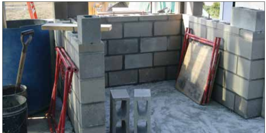
Basic supporting structure of pizza oven.
